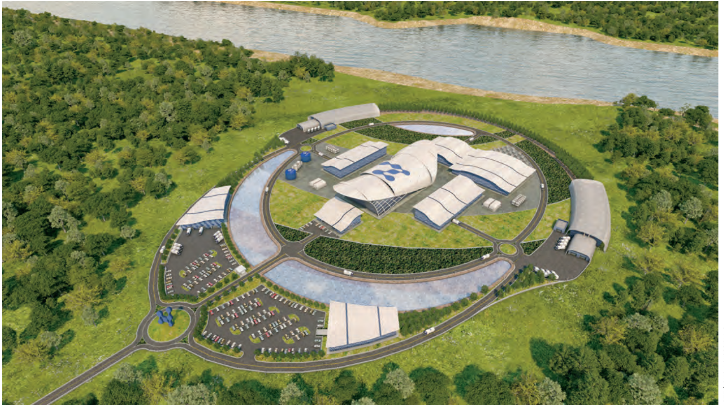
The center building houses 12 reactor modules.
